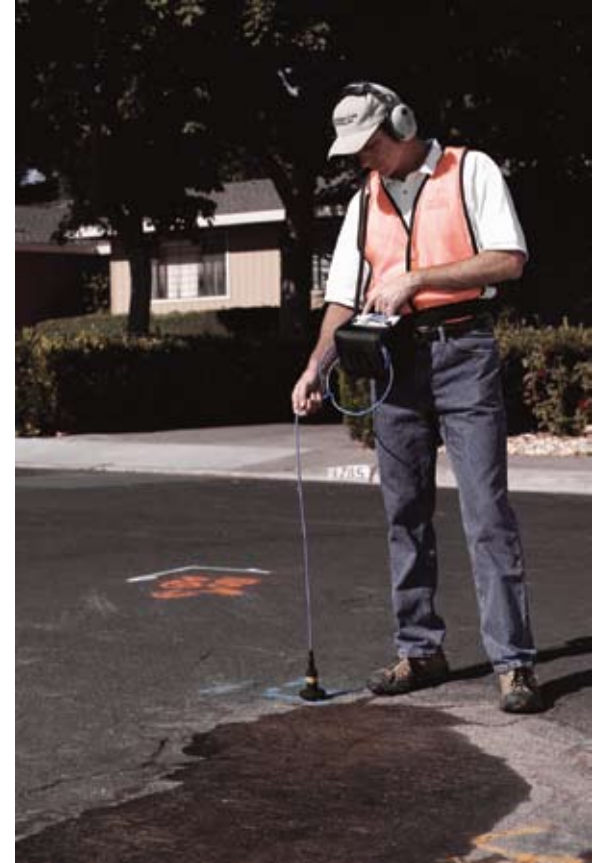
Pinpointing directly over the pipe with the LD-15's base plate
